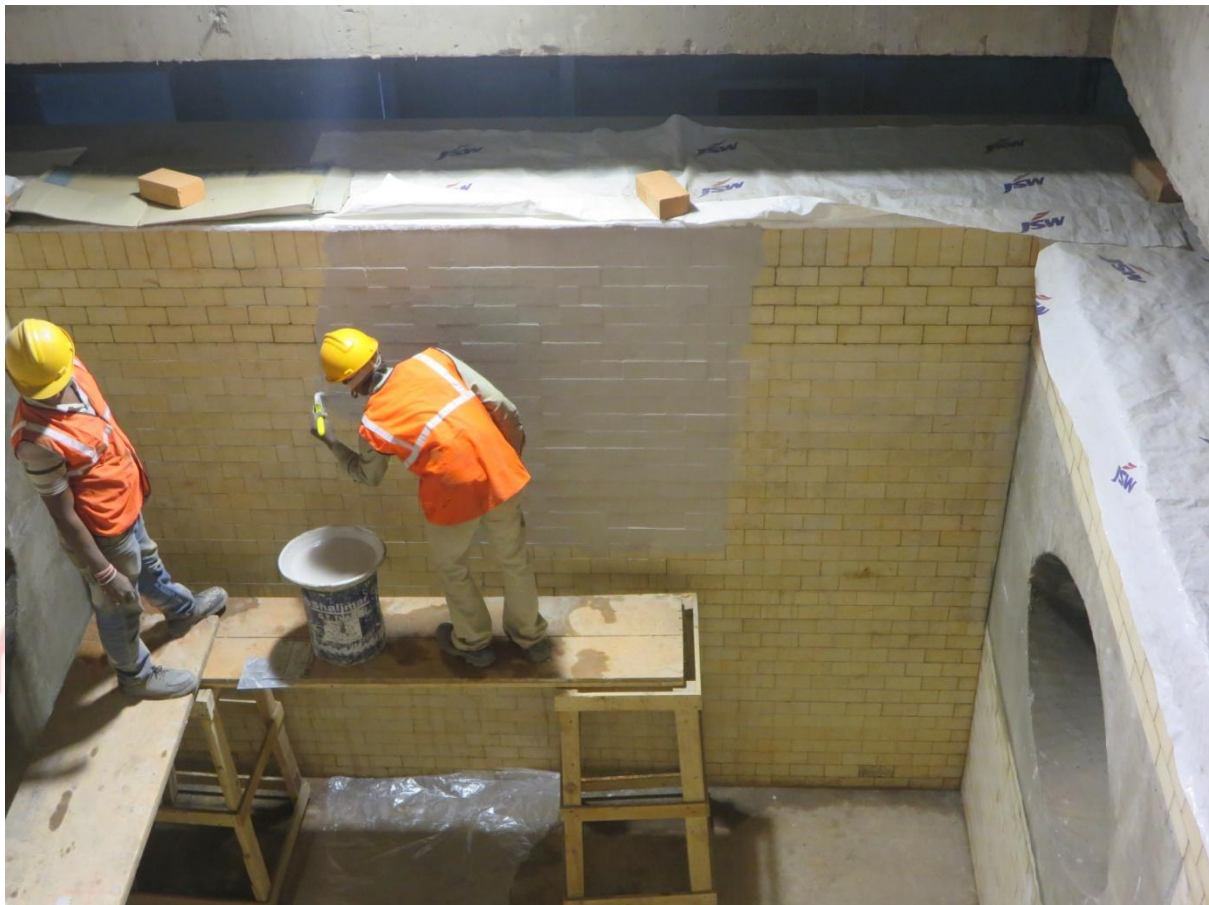
Image 11: Special Coating being applied to the Side Walls of the Pot
