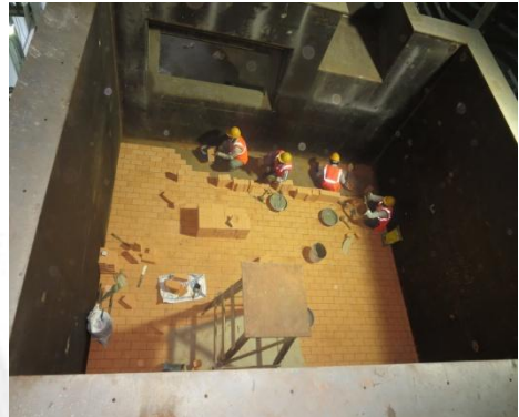
Image 2: Brick Lining of the Bottom of the POT
