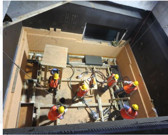
Image 5: Casting of the Outer Layer of the POT
