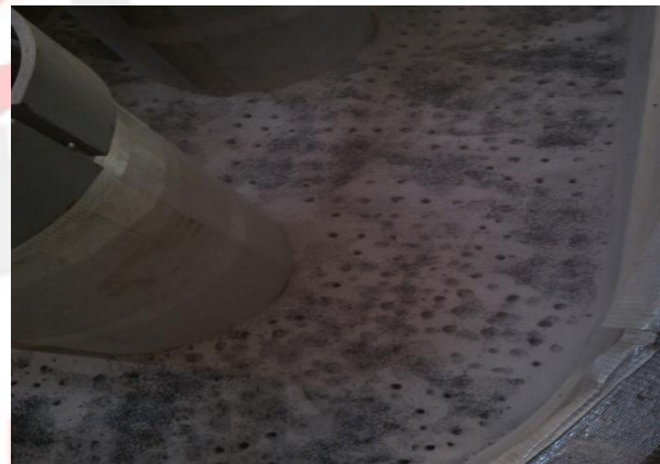
Image 13: Dry Ramming of the Castable inside the Inductor
