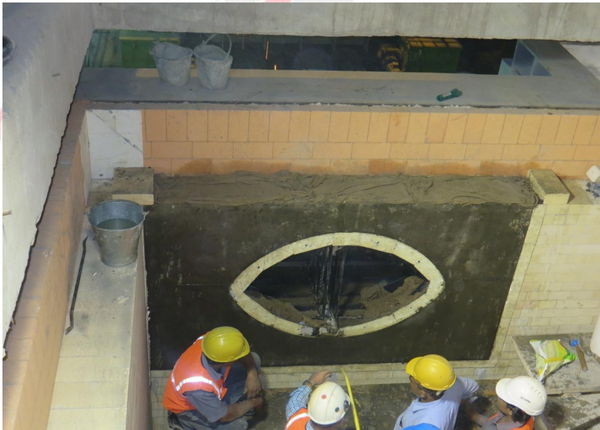
Image 10: Completed Casting of the 2 nd Throat
