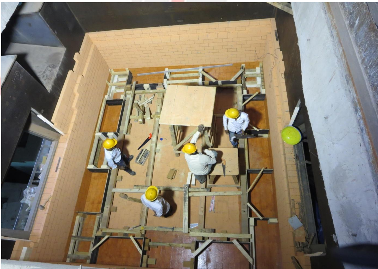
Image 4: Shuttering for the Outer Layer
