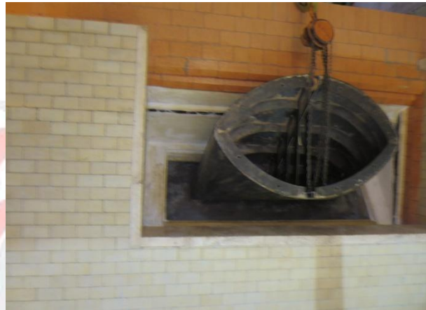
Image 9: Farma Fixing for the Throat Casting
